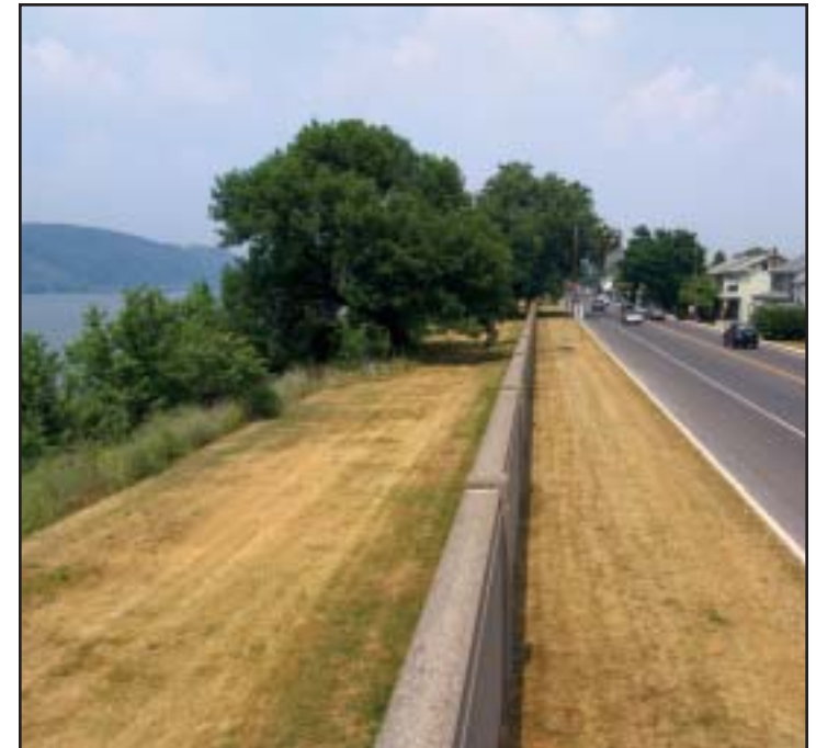
Flood wall along Front Street.
